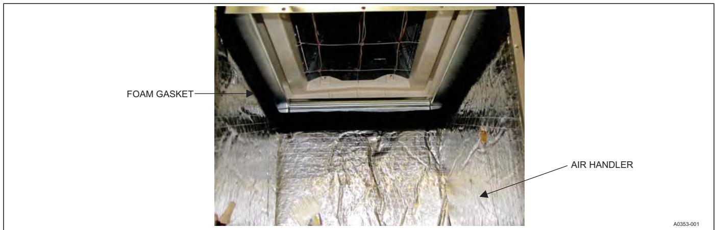
FIGURE 4: Gasket Location
